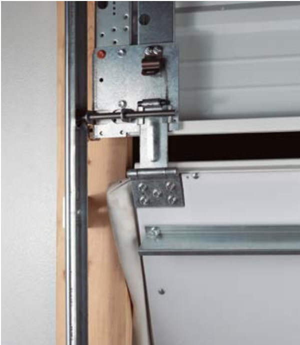
Inside View of Single Bottom Section
